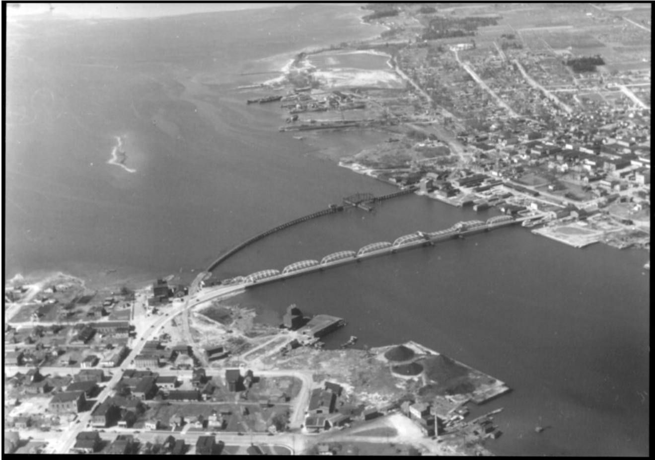
From west side looking east and north, circa early 1940s: The Teweles and Brandeis Grain Elevator (at lower center, with intact dock), the first structure south of the Michigan Street Bridge, stood on the west waterfront of Sturgeon Bay from 1901 through March of 2018. Courtesy of the Door County Historical Museum.
