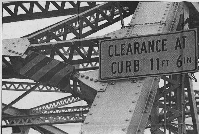
Even before the Michigan Street Bridge is rehabilitated, if it ever is, the state could make truck travel on the span safer by removing the 'portals,' according to bridge engineer Abba Lichtenstein. Portals are diagonal steel brackets (shown here marked with a striped warning sign) that connect the sides to the overhead beams. They serve no structural purpose, Lichtenstein said.
