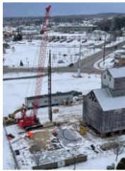
Drilling and placing 51 pilings for support.
