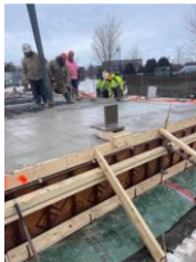
Pouring the foundation.
